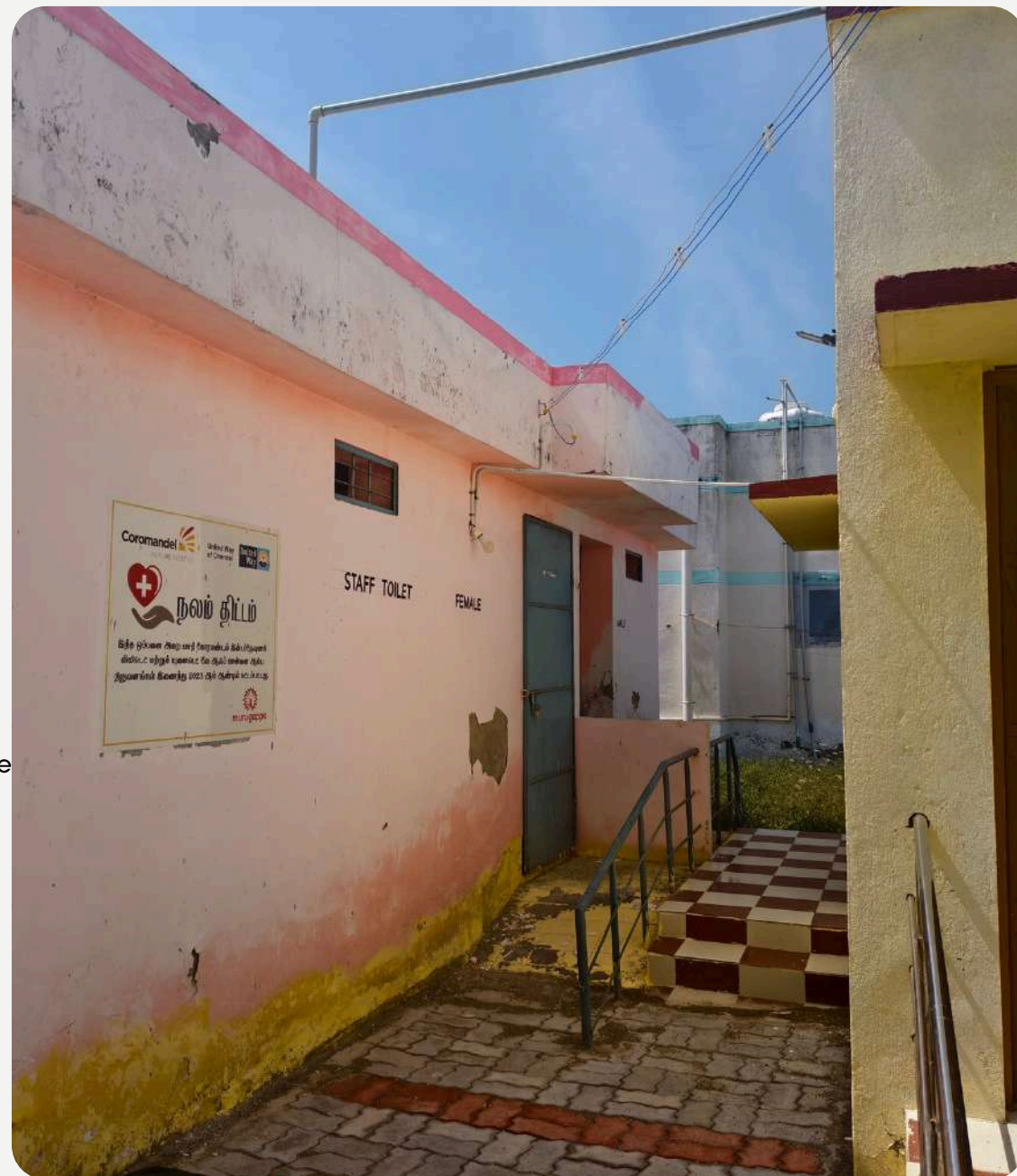
Image 11: Toilet building constructed under Project Nalam - Sholandur PHC, Ramanathapuram
