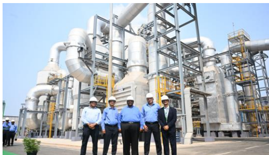
Sulphuric acid plant, Kakinada Commissioning in Q4FY26
