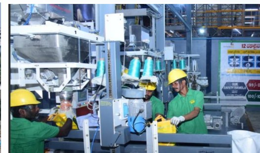
SND Expansion Bentonite Sulphur plant
